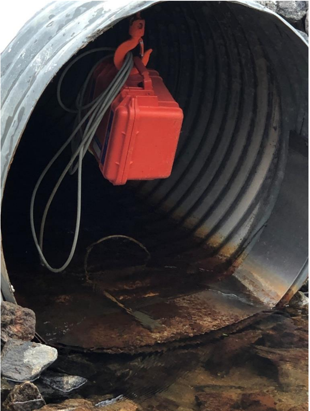
Photo 12 - Instrumentation detail at North Spur
