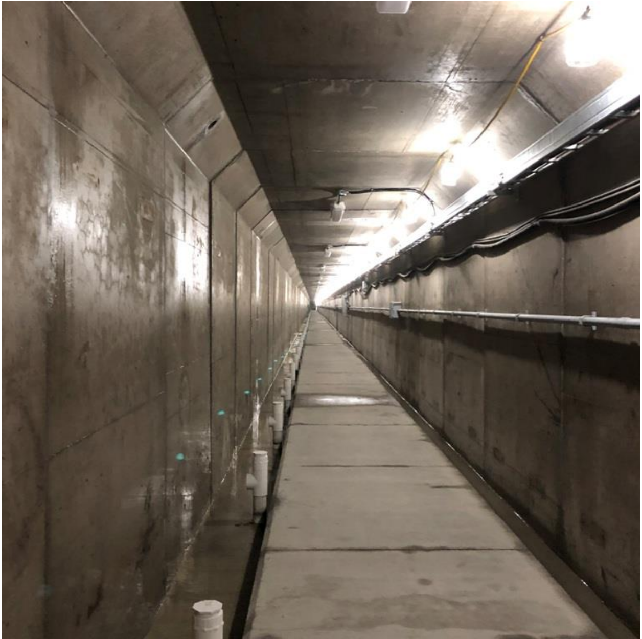
Photo 10 – North (RCC) Dam drainage gallery
