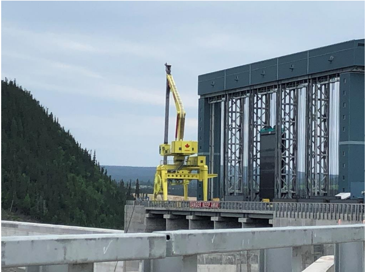
Photo 3 – MF Spillway Hoist Support Structure and Gates
